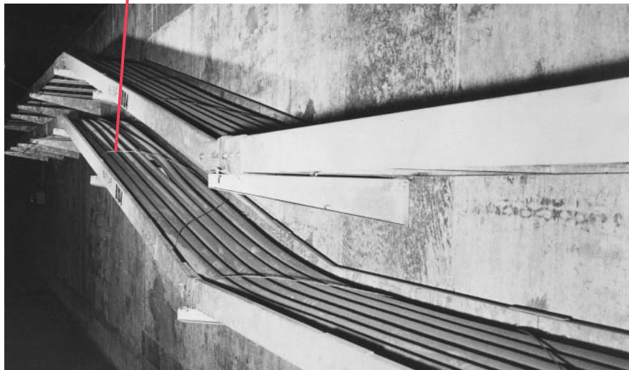
Photo taken at: Bethlehem Steel Corp. Burns Harbor Plant Burns Harbor, Indiana, U.S.A.
